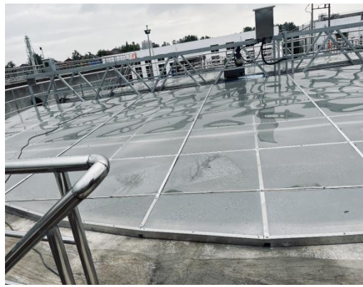
浓缩池加盖密闭
